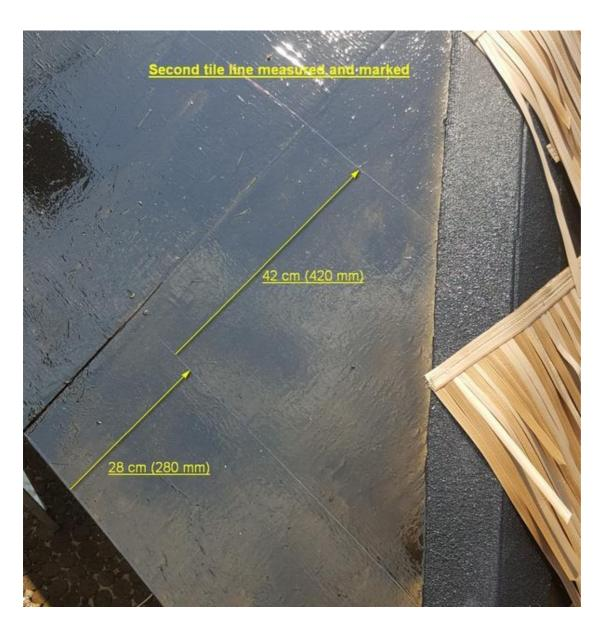
The First line of tiles on the roof edge can now be installed using the recommended Staple method. Pneumatic staple guns or spring loaded handheld staple guns can be used to do the application. The first line of tiles is installed with the bottom section of the Fiber Palm Econo tile protruding past the roof edge. The second bottom rib of the tile is stapled onto the roof edge with the upper bottom rib following the first horizontal line on the roof spaced 28 cm (280 mm) from the roof edge.
