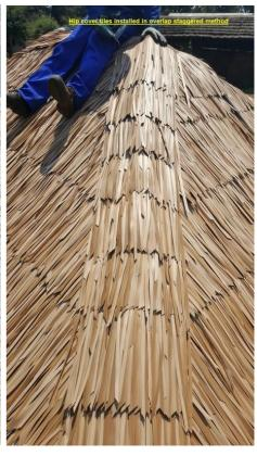
The Hip tile installation is very similar to the traditional method used when installing natural palm leaves on roofs and covering the hips. T method is also synonymous to the clay tile hip cover installation method used on clay tile roofs.
