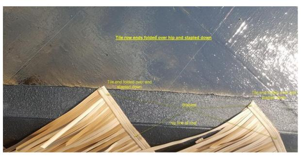
As can be seen in the photo below once the Fiber Palm Econo tile rows have been installed and folded over the hips as specified a diamond pattern of exposed waterproofing will be visible running along the hips on the roof. This will be covered but he installation of the Half Fiber Palm Econo tiles that will be applied over the hip section.
