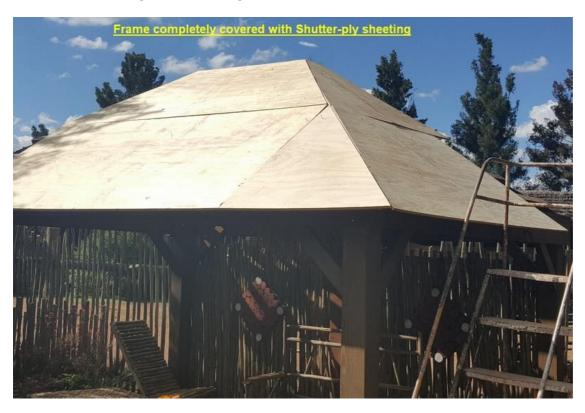
Once the Shutter-ply has been installed the exterior of the shutter-ply is waterproofed with Fiber Dual component waterproofing.
