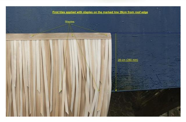
Once the first row of tiles has been applied and stapled down the second row of tiles can be applied in the recommended specified manner, spaced 42 cm (420 mm) above the first line of tiles to rib. The second line of tiles will overlay the first row of tiles as will every following row overlapping the previous row of tiles. The Fiber Palm Econo tile will have distinct even horizontal lines on the exterior of the roof once installed.
