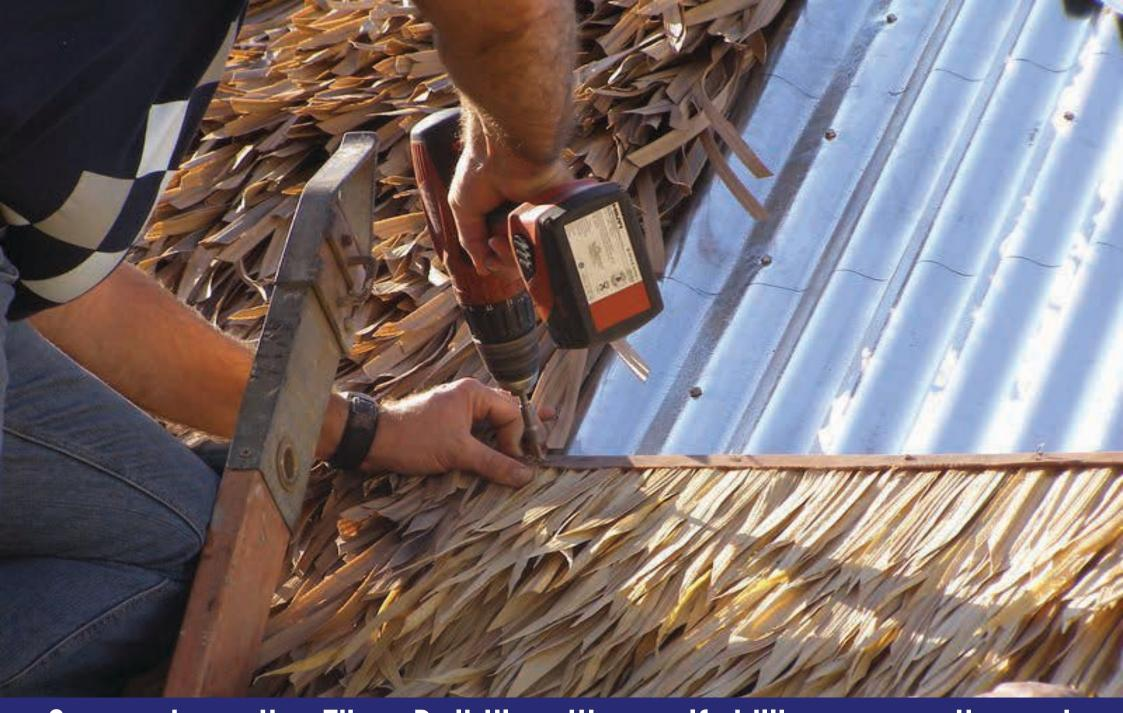
Screw down the Fiber Bali tile with a self drilling screw, through the polyurethane backing strip of the tile.
