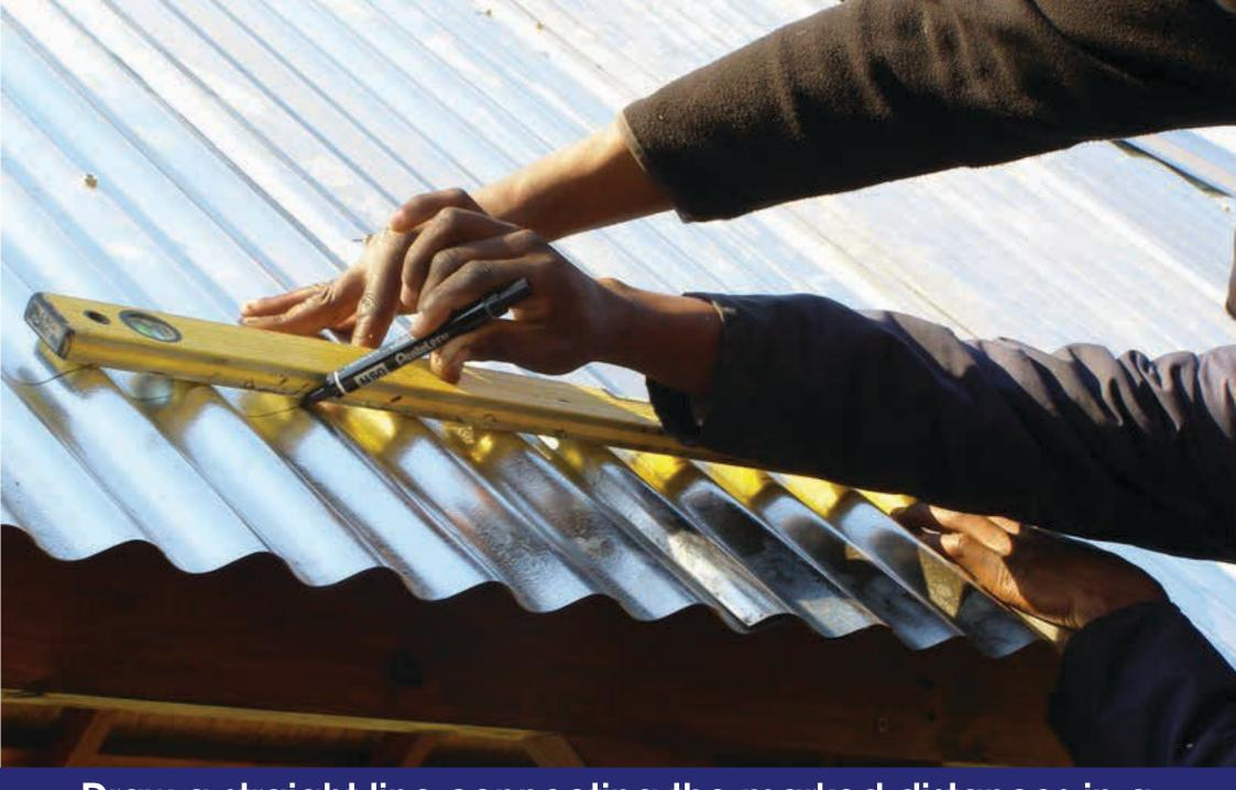
Draw a straight line connecting the marked distances in a solid line
