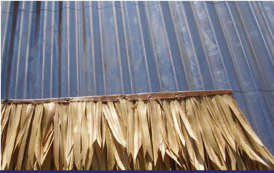
Screw the first tile down onto the metal sheet roof with self-drilling screws
