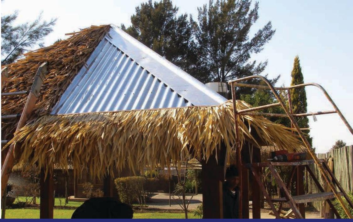
Continue the first line on the roof edge until completed, this will lay the foundation for the installation.
