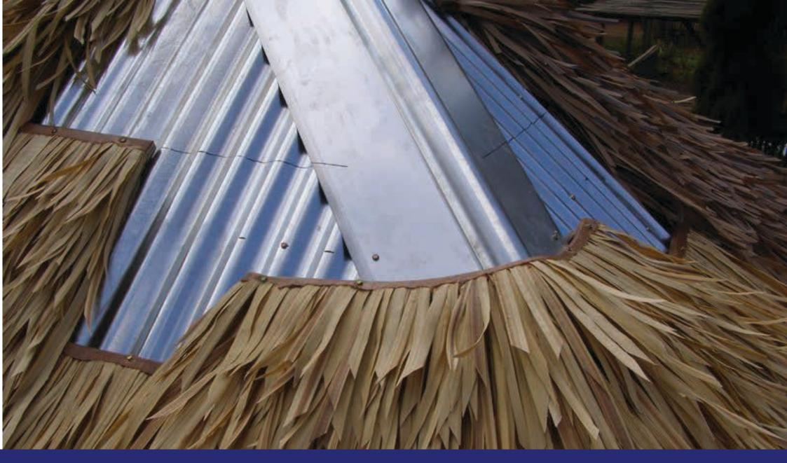
An additional Fiber Bali tile is fitted half way between the drawn lines on the roof on the hips to ensure that an even thickness is maintained.
