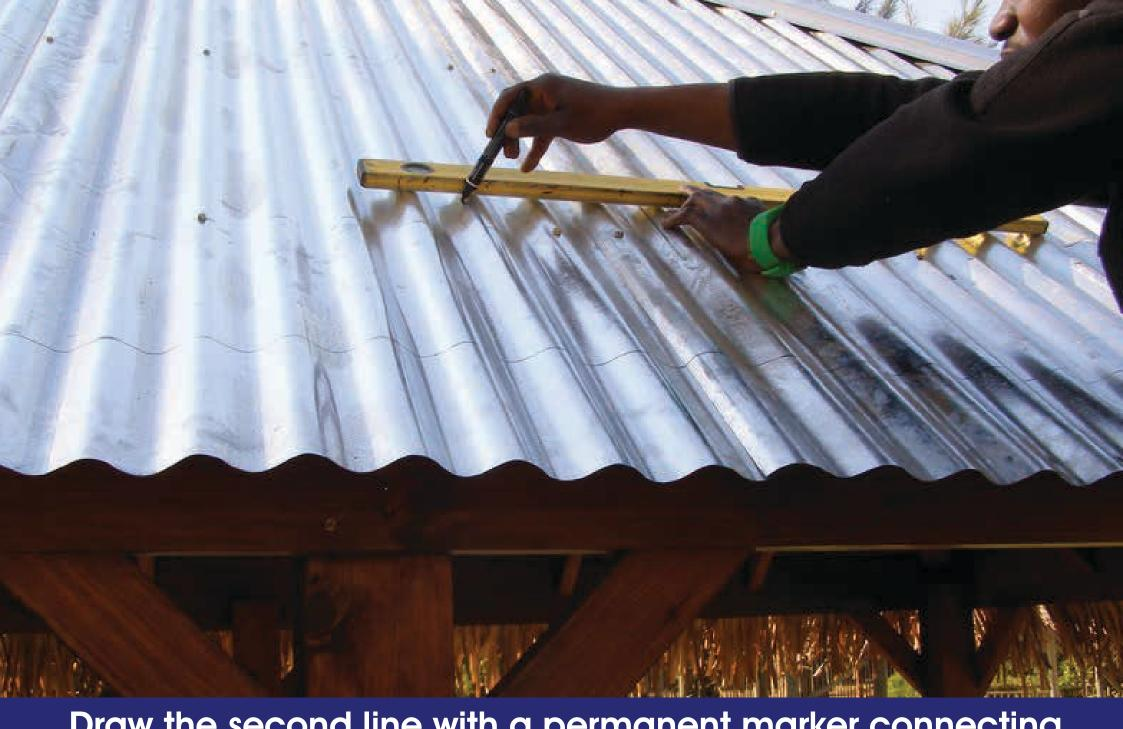
Draw the second line with a permanent marker connecting the 400mm marks in a solid line
