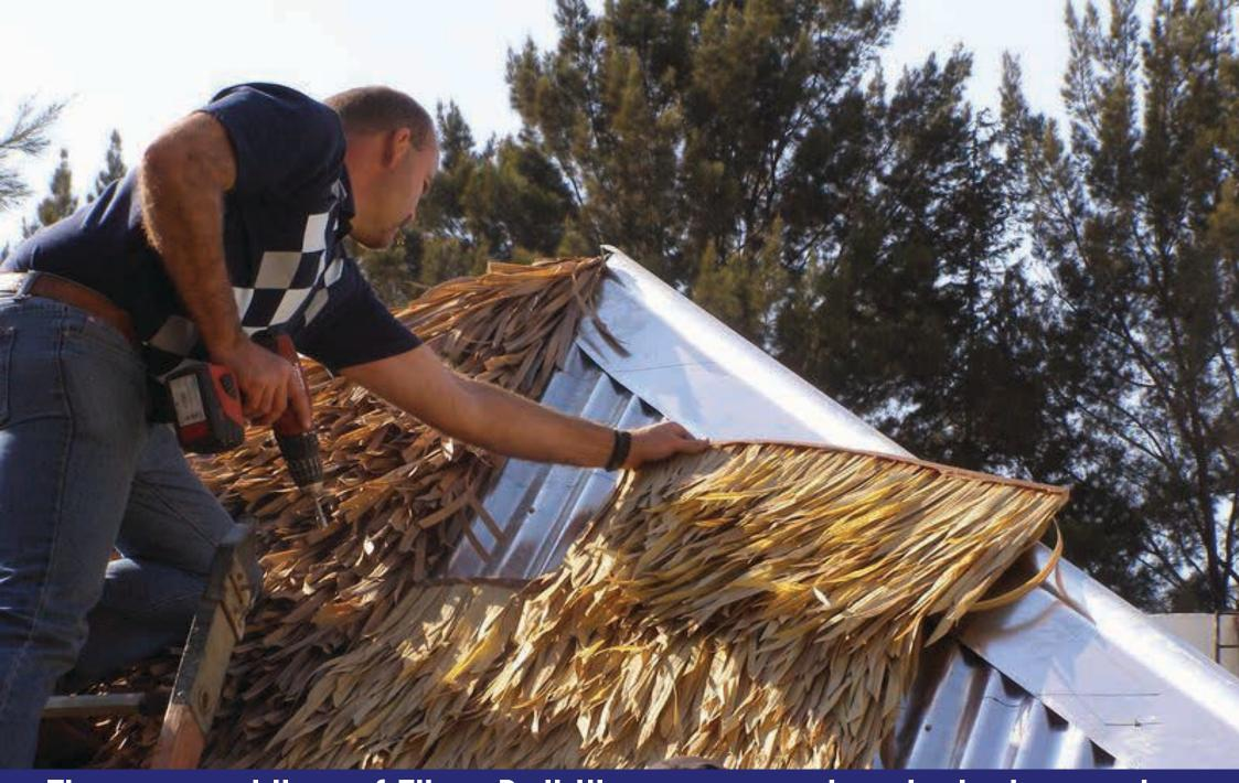
The second line of Fiber Bali tiles can now be started, ensuring to line the Polyurethane to the drawn line on the sheet roof.
