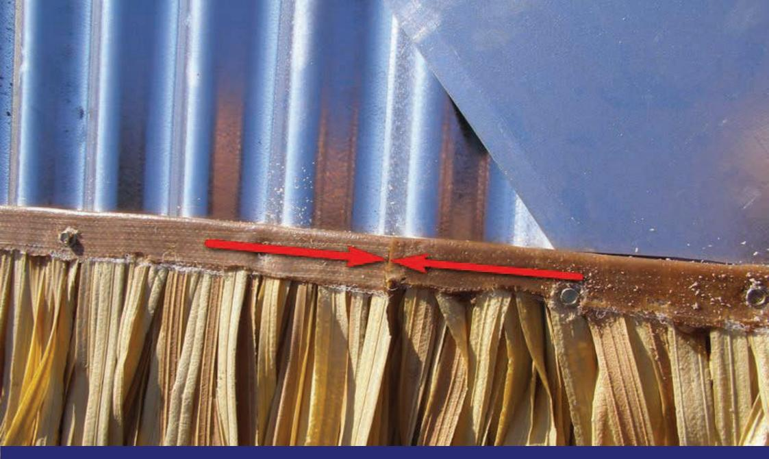
But up the polyurethane of the following tile to the polyurethane of the previous tile and screw down ensuring to a line to the drawn line on the roof.
