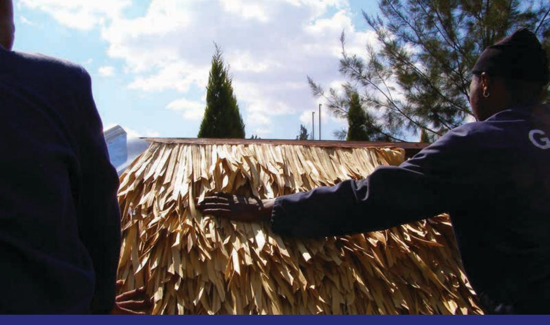
The simple installation process is continued until the apex of the roof is reached. Ensure that tiles are installed right up to the apex for the best finish.
