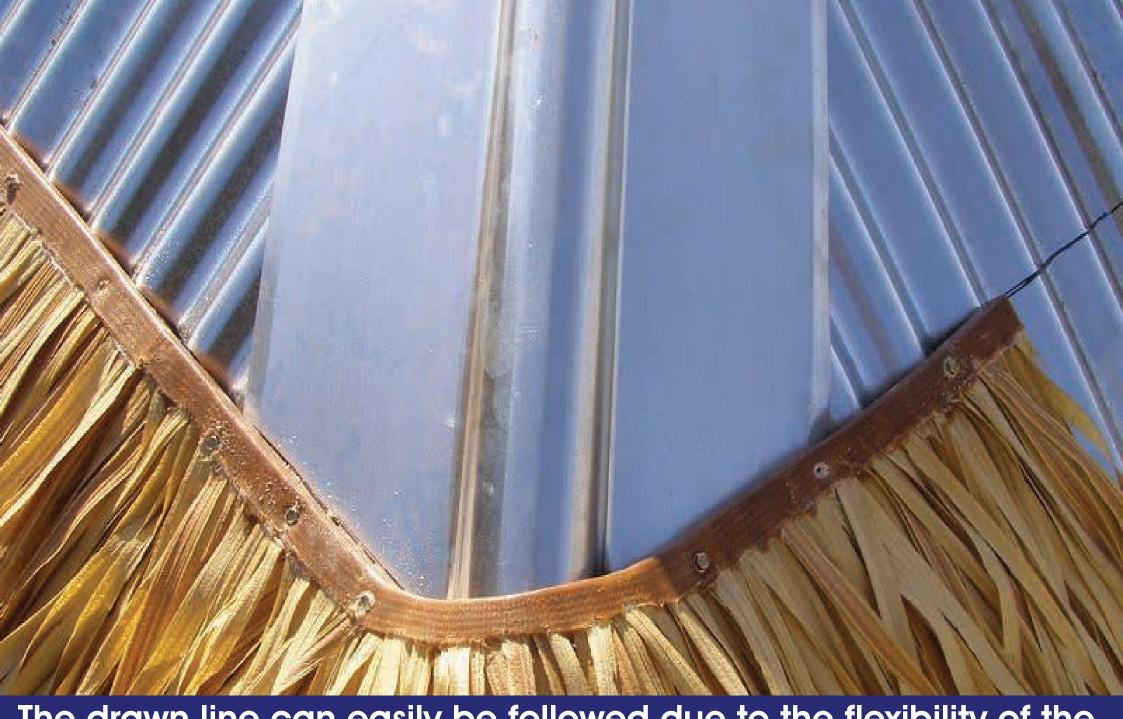
The drawn line can easily be followed due to the flexibility of the polyurethane backing strip of the Fiber Bali tiles.
