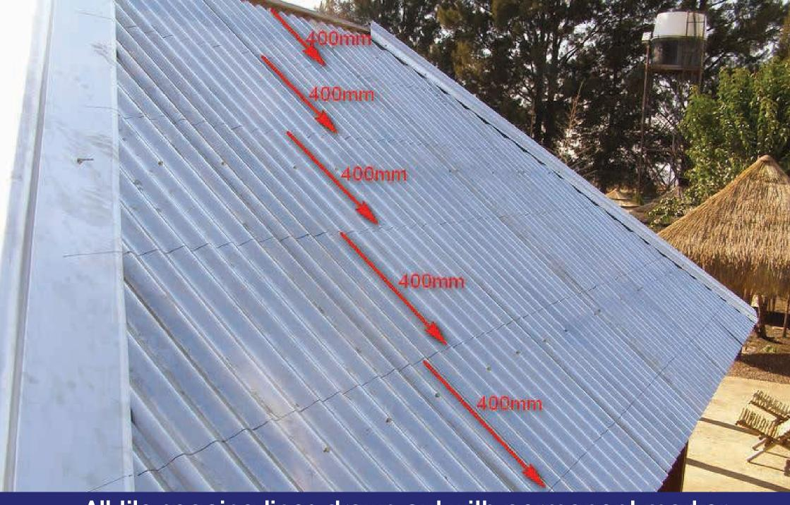
All tile spacing lines drawn out with permanent marker on sheet roof
