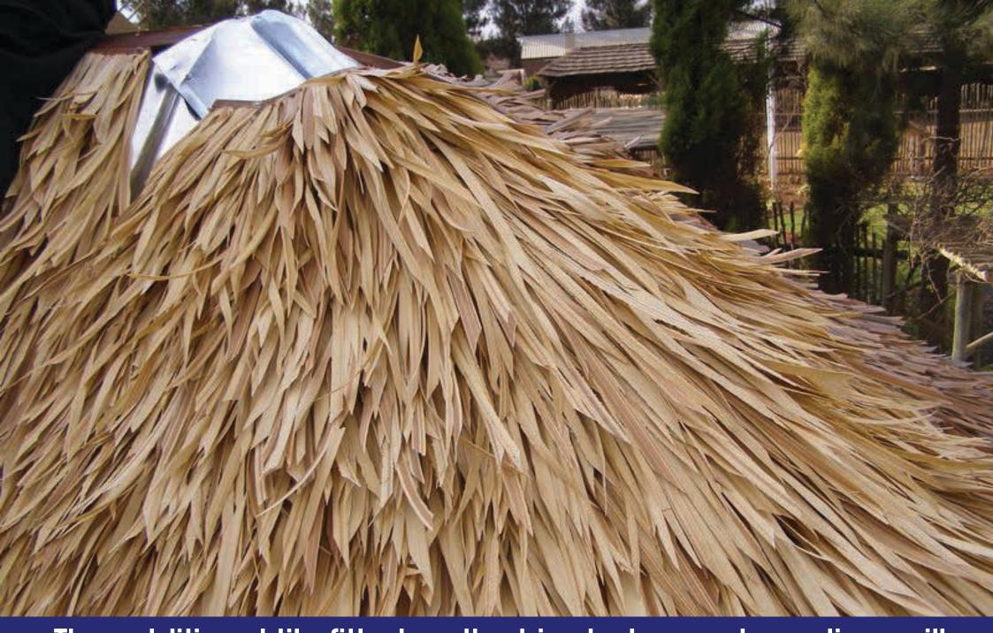
The additional tile fitted on the hips between drawn lines will ensure a perfect even cover matching the rest of the clad roof.
