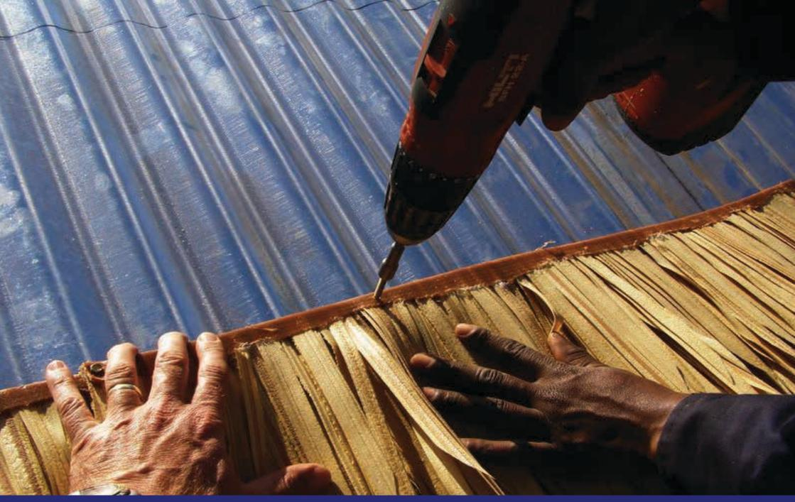
Screw down the tile by ensuring the screw enter the sheet roof on the raised section also called the rise.
