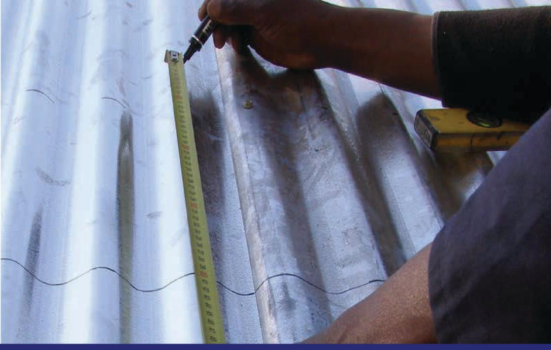
Mark the second line spaced 400mm from the first line drawn close to the roof edge
