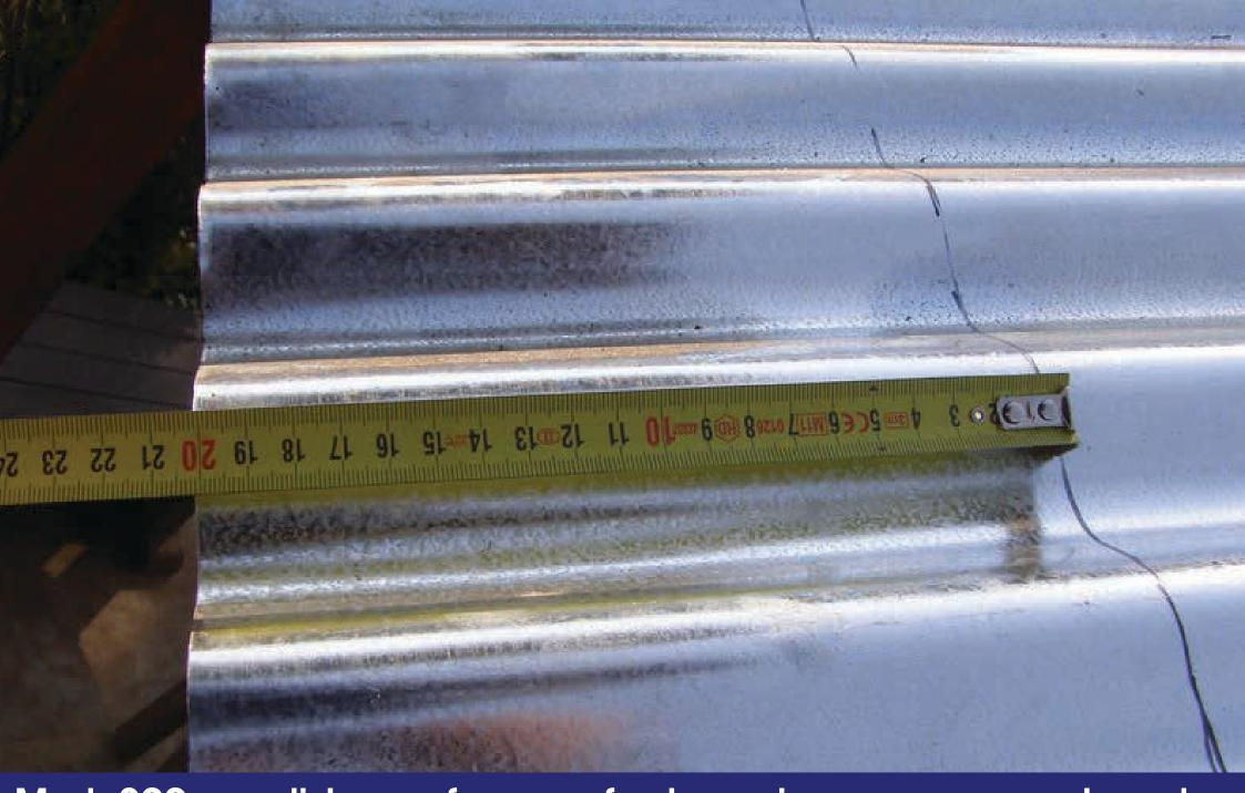
Mark 200mm distance from roof edge using a permanent marker and a tape measure
