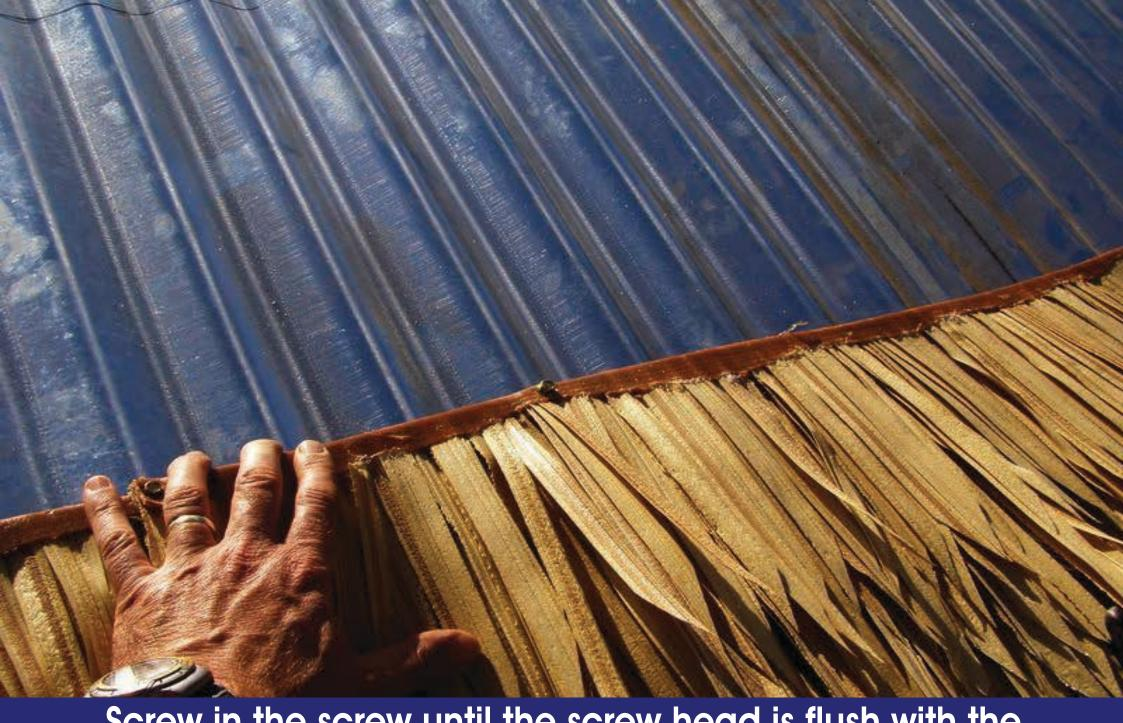
Screw in the screw until the screw head is flush with the polyurethane backing strip of the tile
