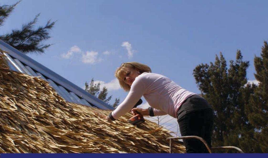
No special skill is required and anybody can do the Fiber Bali installation on metal sheet roofing as long as the aforementioned guidelines are followed.
