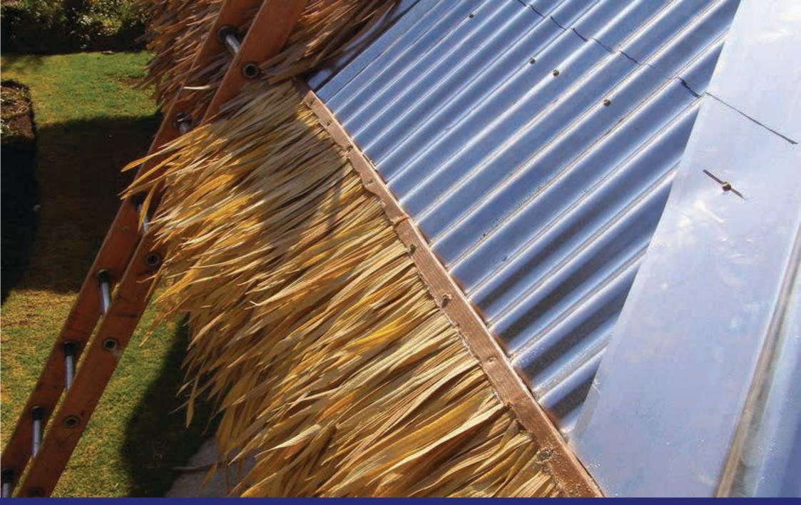
Follow the drawn line on the metal roof aligning the tile backing with the drawn line
