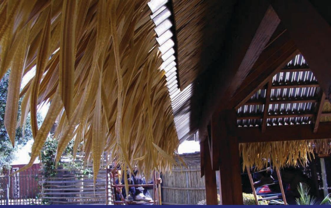
The first line of Fiber Bali tiles will provide a fantastic drooping finish over the roof edge of the sheet roof
